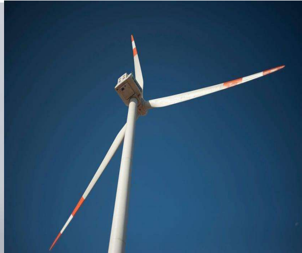
Horizontal axis wind turbine
